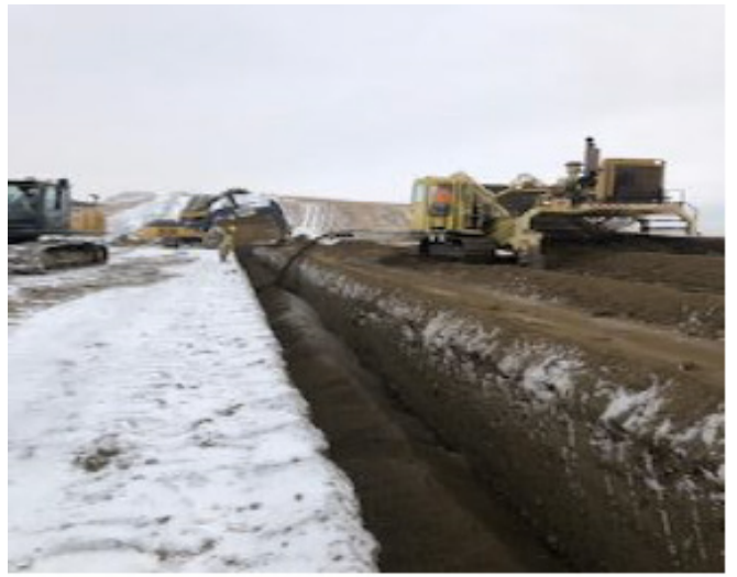
Shading mainline – km 220+980 – Nov 3, 2018
