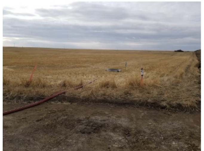
Discharge hose for pumping water– km 175+250 – Oct 30, 2018
