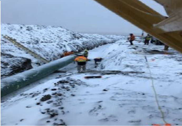
Tie-in weld - km 175+073 – Nov 3, 2018
