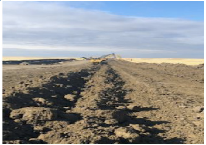
Shading crew pulling soil– km 209+200 – Oct 30, 2018
