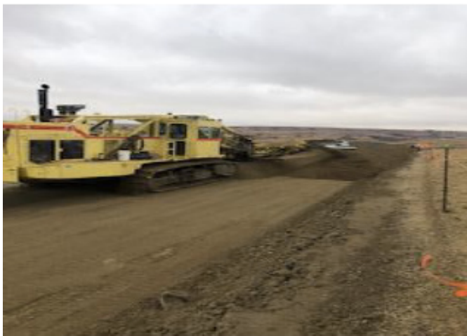
Ditcher digging in Heritage area – km 259+100 – Nov 1, 2018
