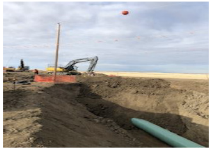
Excavator shading pipe – km 213+300 – Oct 31, 2018
