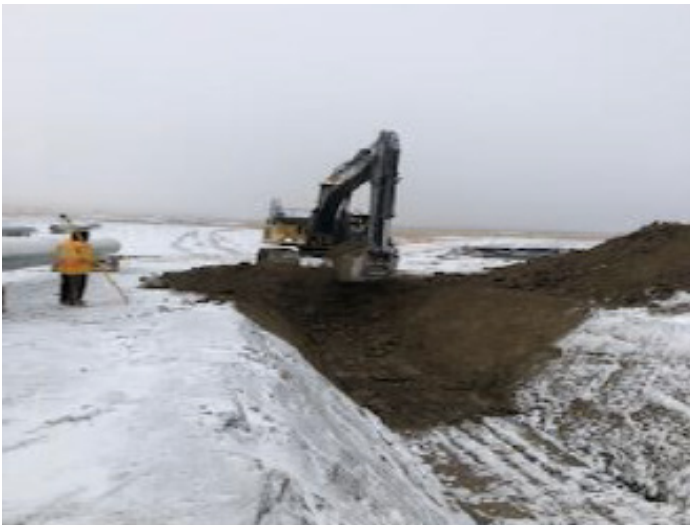
Digging bell hole in Heritage area- km 222+275 – Nov 3, 2018
