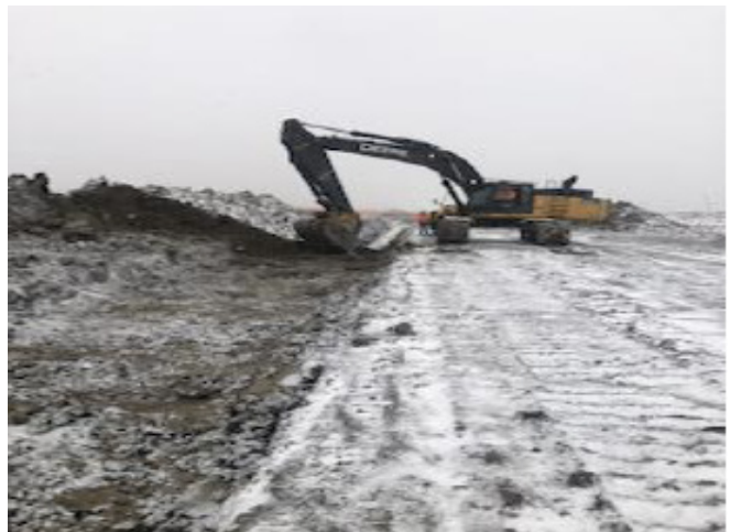
Backfill crew shading – km 182+172 – Nov 2, 2018
