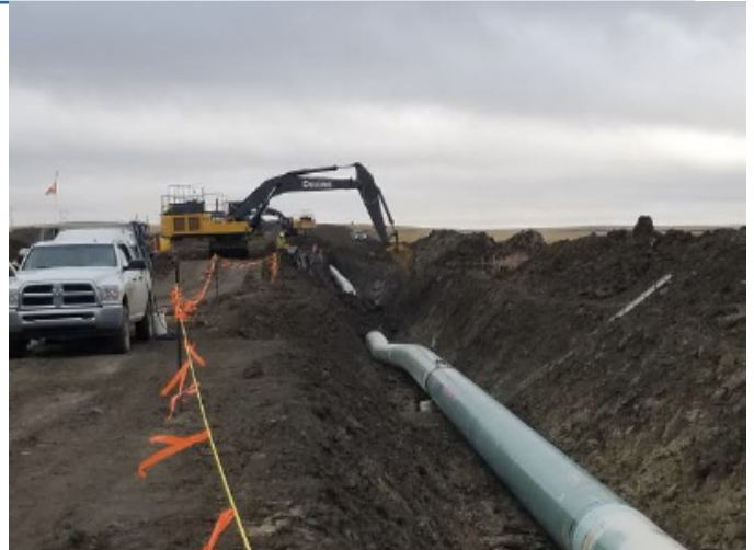
Shading and backfill tie-in– km 195+200 – Nov 1, 2018
