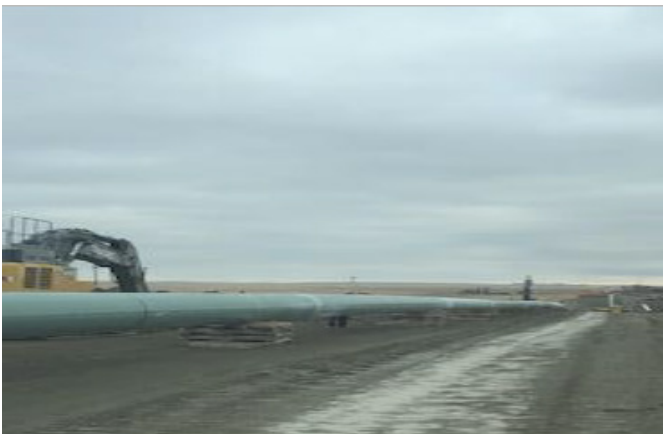
Excavators digging mainline ditch – km 210+900 – Oct 29, 2018
