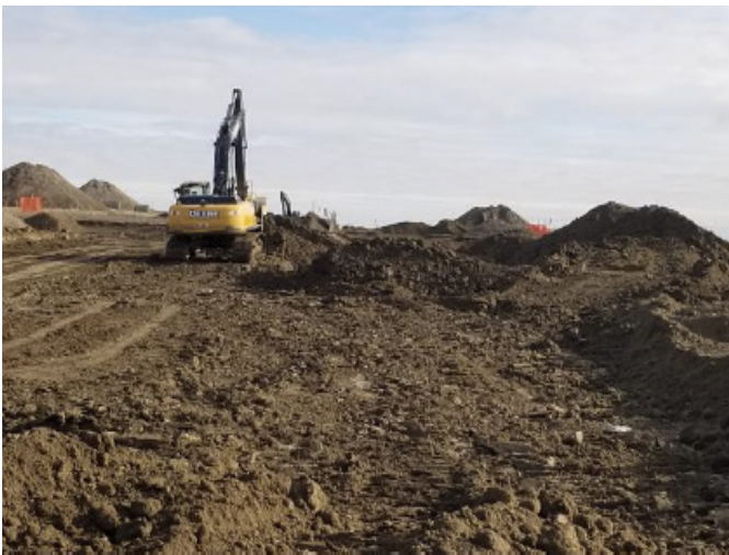
Backfill tie-in – km 171+600 – Oct 30, 2018
