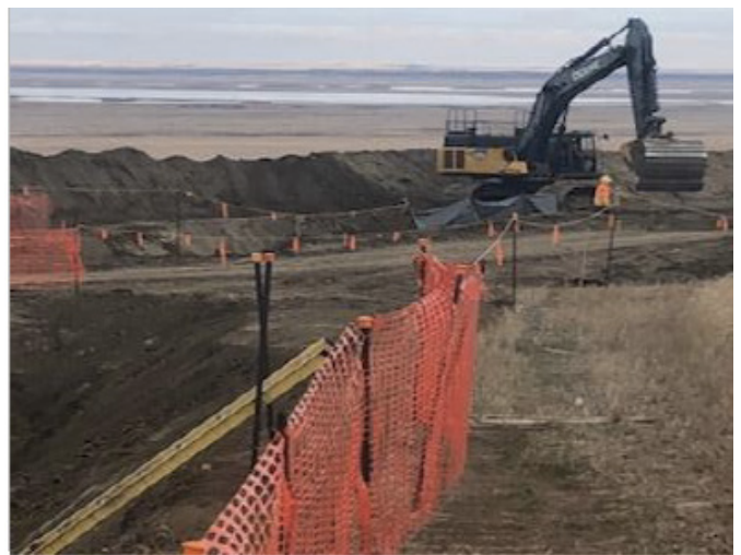
Excavator digging bend for tie-in– km 172+140 – Oct 30, 2018
