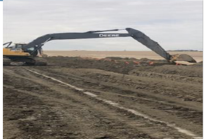
Excavator shading pipe – km 213+300 – Oct 31, 2018
