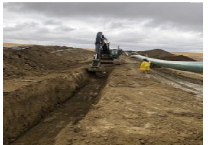
Excavator digging on the west side – km 219+415 – Nov 1, 2018
