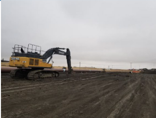
Pulling bore– km 196+000– Nov 1, 2018
