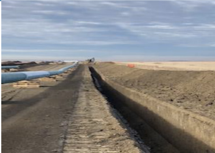
Ditch before lowering in – km 218+900 – Oct 31, 2018
