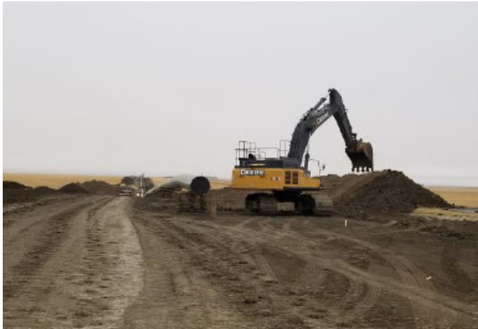
Excavator digging ditch in Heritage area - km 222+300 – Nov 2, 2018
