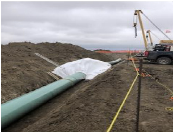
Final tie-in weld – SF 113 – Nov 1, 2018
