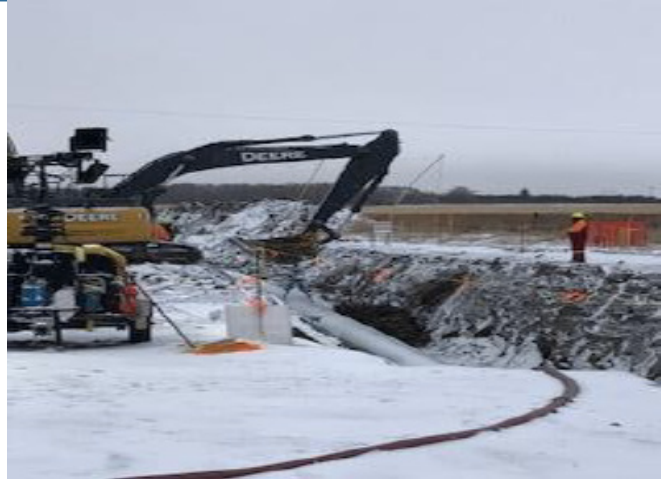
Excavator shading pipe in wetland – SF 110 – Nov 3, 2018
