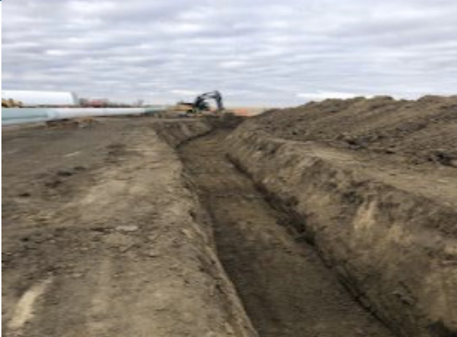
Excavator digging out bends in mainline ditch– km 211 – Oct 30, 2018
