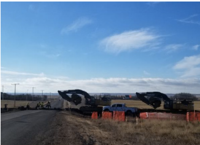
Crossing equipment – km 209+789 – Oct 29, 2018
