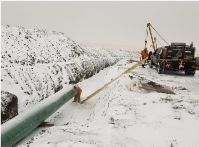
Prepping pipe for tie-in - km 193+050 – Nov 3, 2018
