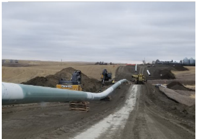
Digging ditch– km 211+100 – Oct 29, 2018
