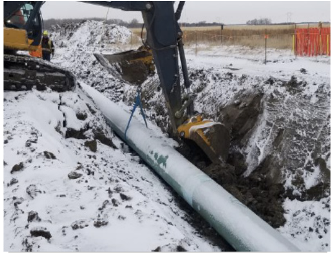
Shading tie-in section – km 182+100 – Nov 3, 2018
