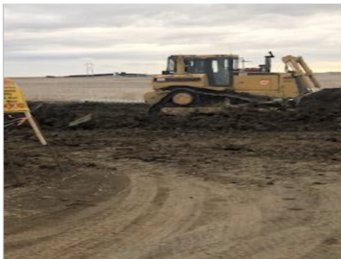
Dozer pushing clay– Km183+007 – Oct 30, 2018
