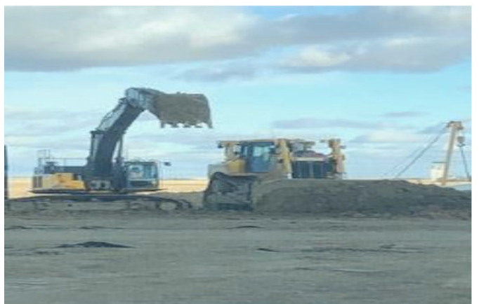
Excavator digging ditch – SF 120 – Oct 29, 2018
